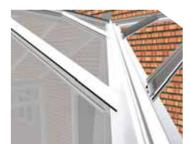
Glaze the first panel either side of the valley at the ridge wall plate intersection. Silicone seal the void at this intersection, continue glazing either side of the valley.
