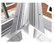
The valley assembly should now be aligned at the ridge, wall plate and eaves beam with the fixing bolts. Secure the valley wings using M6 nuts.
