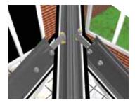
Align the jack rafter with the hip bar, ensuring the correct position is obtained on the glazing bar at 90° to the eaves beam.
