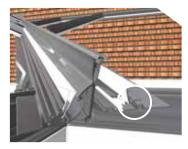
Prior to fitting the glazing bar top caps the glazing trim should be fitted to each valley wing. (the picture shows the section with no glazing for clarity) Apply a bead of silicone on the top inside edge of the glazing trim and push into place.
