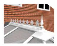
Complete lead flashing over the ridge flashing trim prior to glazing the wall end panels.
