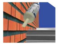
Seal the end of the eaves beam using low modulus silicone prior to fitting the next section.
