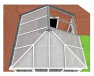
The glazing panels supported by the hip bars should be glazed first, thus enabling the sealing of the radius end without climbing on the roof. Jack rafter top caps should be sealed to the hip bars at this point using low modulus silicone.
