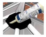
Apply a bead of silicone around the outer edge of the foam weather seal following the profile contours.
