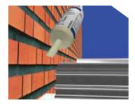
Seal the profile end of the eaves beams using low modulus silicone prior to fitting the next section.
