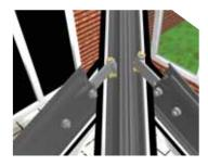
Fully tighten the jack rafter arm and the pivot bolt nut.
