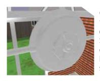
Cover the aluminium tie bar ring with the circular covers provided. Seal the M10 nuts on the external face of the eaves beam with a low modulus silicone.
