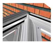
On roofs with valleys, the valley should be fitted after the ridge and wallplate have been fitted and supported. This is before all the glazing bars are fitted.
