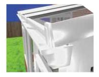
Located front edge of the gutter onto the gutter brackets and rotate upwards into the gutter bracket. Continue process on all sides.
