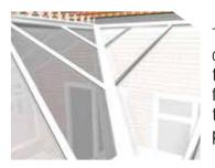
The external valley top cap can now be fitted along the valley section. Finally fit the valley end cap using the screws and cover caps provided.
