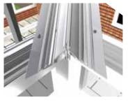
Prior to fitting the aluminium valley sections it is necessary to seal along the eaves pivot where the valley sits using a low modulus silicon.
