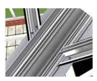
Start locating the glazing bars between the ridge and valley again using the M6 bolts provided.
