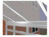
Fit the internal eaves beam covers to the eaves beam.
