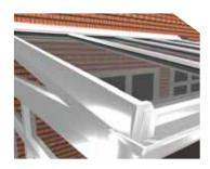
Fit the wall end bar cloaking trim, the eaves beam and the wall plate end caps (if required).
