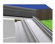
The glazing retainer should be inserted within the eaves pivot between the glazing bars. Complete the glazing sequence as with the polycarbonate method. You will note the glazing end trim is omitted.
