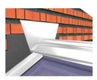
Cut a slot into the brickwork to receive lead flashing above the ridge, using the ridge flashing trim as a guide to the height of this slot.
