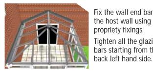
Fix the wall end bar to the host wall using propriety fixings. Tighten all the glazing bars starting from the
